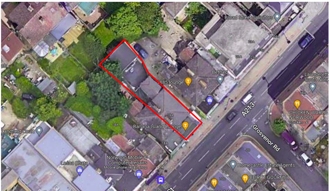
Figure 1: Aerial street view highlighting the application site within the surrounding streetscene
